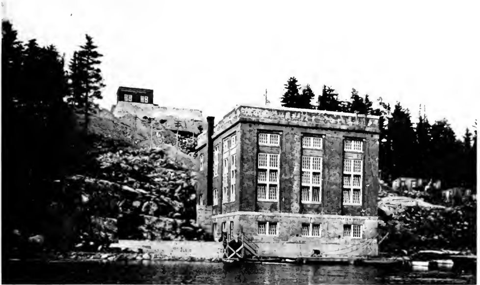
First Unit of Power Plant at Temiskaming, showing Gatehouse and Forebay.
